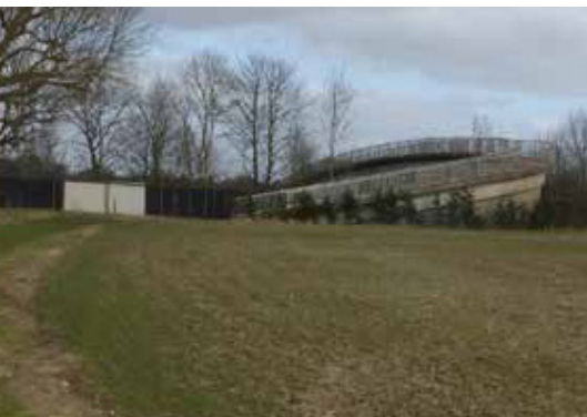
Cantelope Farm - M11 bridge
